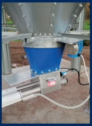
PPP Silo Vibrators come standard with their own control box, meaning less wiring costs for the sparky as it only needs to be supplied power. They also come standard with two proximity sensors for each silo. We use two as there needs to be a sensor over each auger line to make sure it picks up small bridges in the silo.
