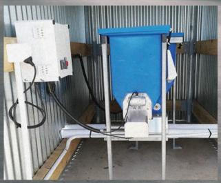
PPP mineral dispensers are designed with ease of use coupled with the knowledge of what works and what doesn't work. This means that the design we have today ensures that there is no bridging of minerals and accurate feeding. They can be used with Powders (such as causmag), Prills, and Pellets.
